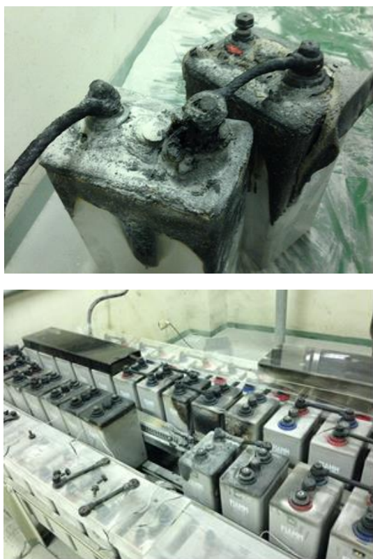
圖 1 蓄電池燒毀事故現場照片。 Figure 1 Field observation of lead acid battery.
