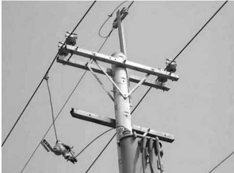
圖1 現場勘查。 Figure 1 Field investigation.
